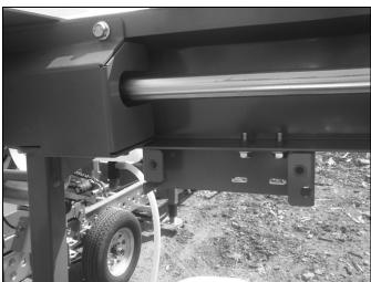
Install the water valve bracket (8) onto the lower part of the rear horizontal cover. Secure it with 3/8 x 3/4" flanged bolts (4).
